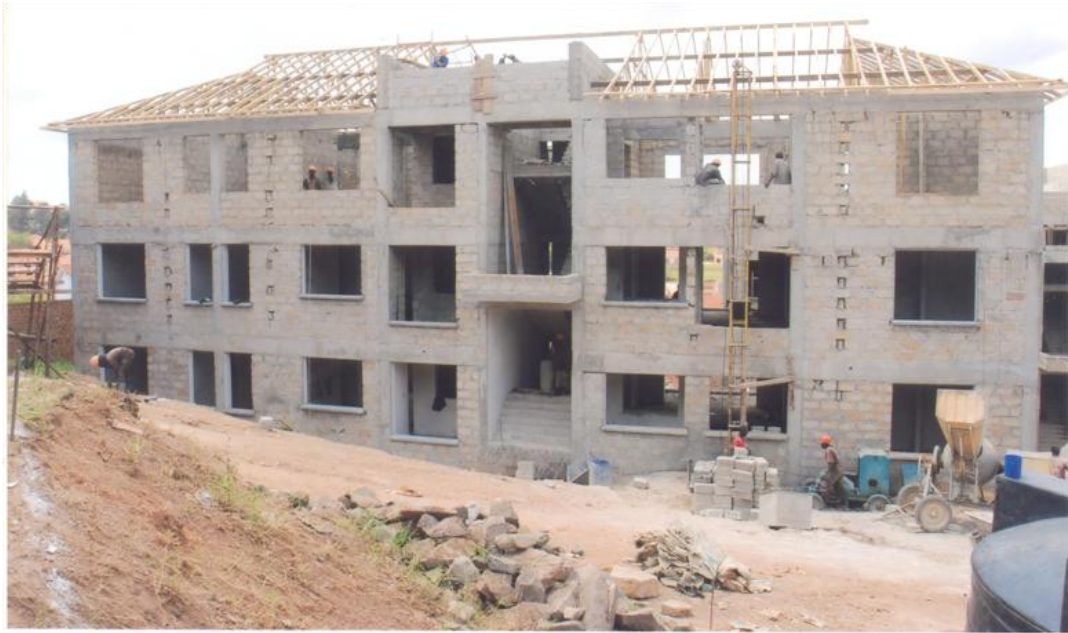
One of UCA's residential apartments being roofed. Site: Plot 47 Bukoto Crescent, Kampala
