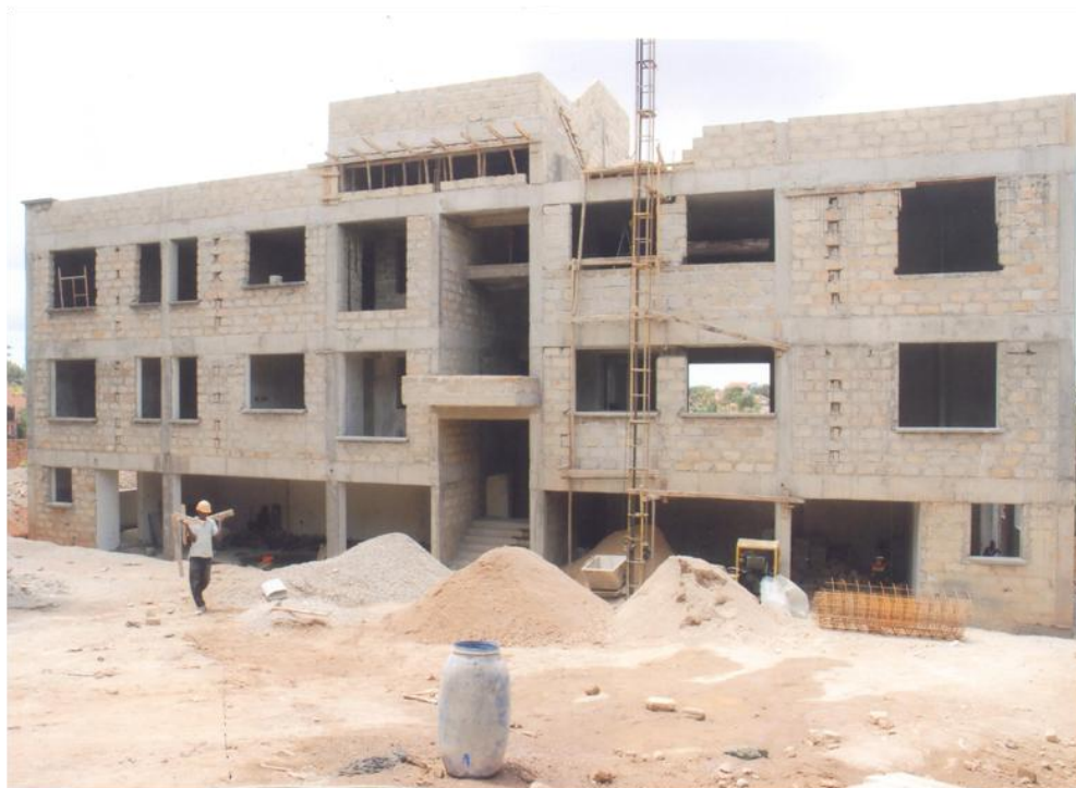
One of UCA's residential apartments almost at the roofing stage. Site: Plot 47 Bukoto Crescent, Kampala
