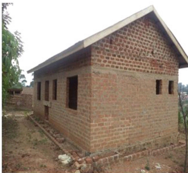
A house at Polysack PHC built using ISSBs
