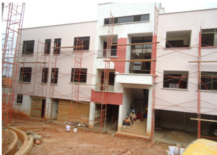
UCA's construction site at Plot 47 Bukoto- Naguru Crescent, Kampala
